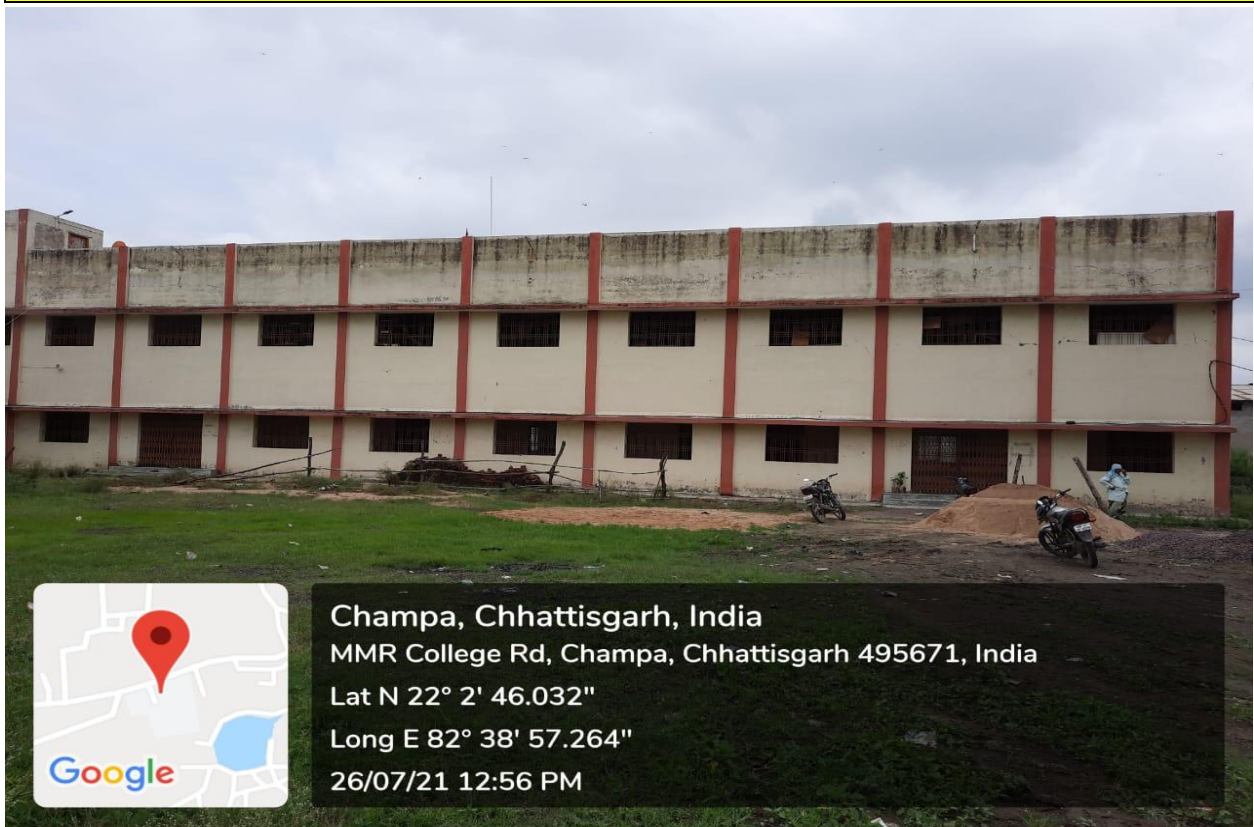
Building from State Govt. Funding 2017
